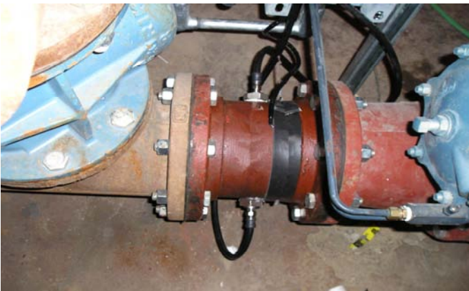
Spool Piece Installed in Plant
